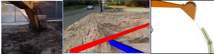
**Figure 11** Visualization of excavator proximity to expected buried utility locations.
