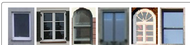
Fig. 6 Window examples from facade images. Windows occur in very different shapes and sizes which complicates the composition of an adequate set of features describing the windows’ characteristics
